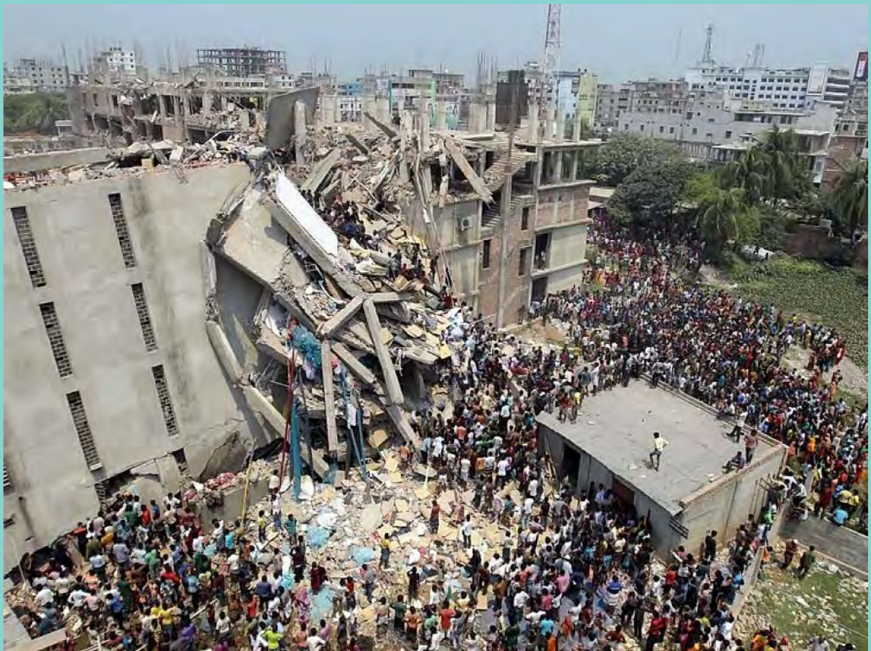
2013 Rana Plaza collapse in Bangladesh
